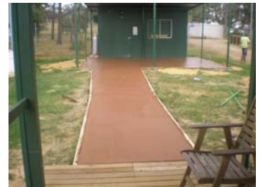
October Concreting of the tea area
